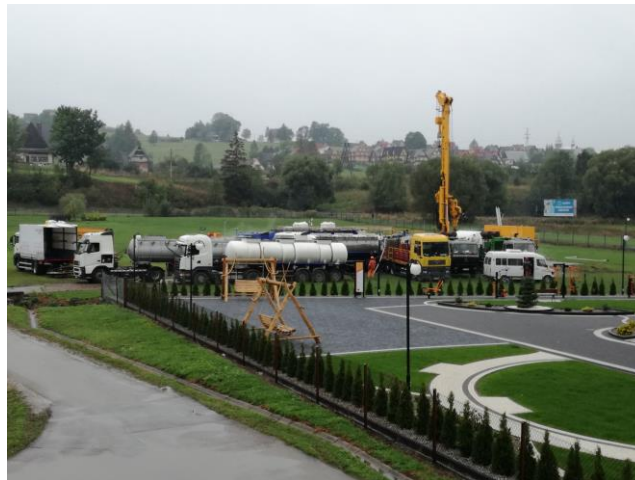
Acidizing works in progress, Bańska PGP-3 geothermal well.
