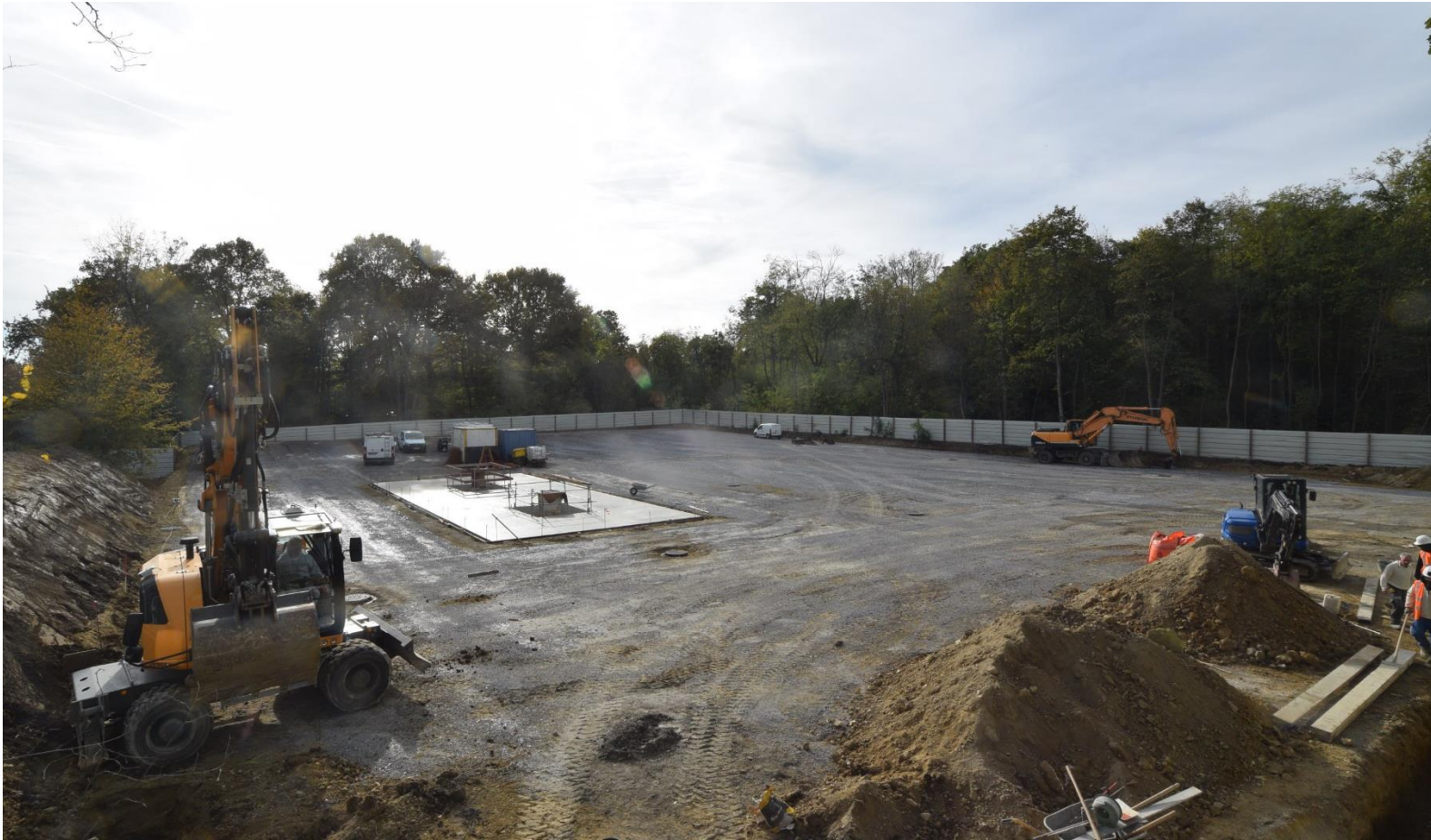
Construction work (28th October 2019)
